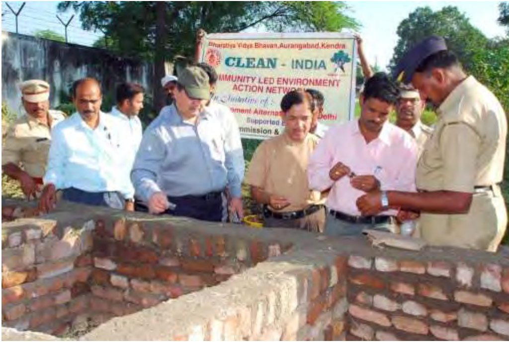
Solid waste disposal
